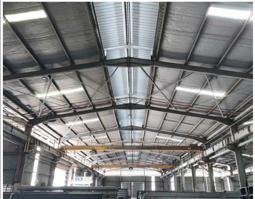
Changing into a transparent roof and installation of LED lights
