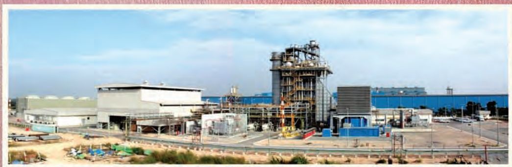
Power Plant at Rayong
