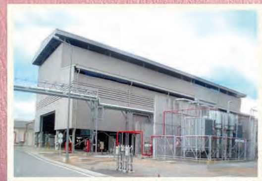
Steam Turbine Generator Set
