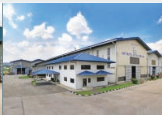
MYCRON STEEL FACTORY
